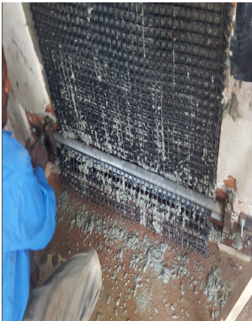
(e) Stretching of textiles by rotating knob
