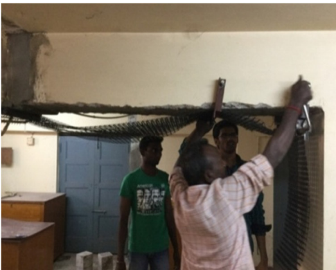
(e) Stretching the textiles by rotating the knob
