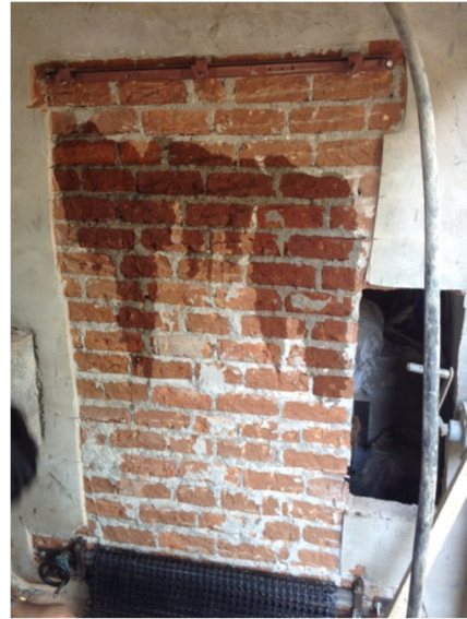
(b) wetting of masonry wall
