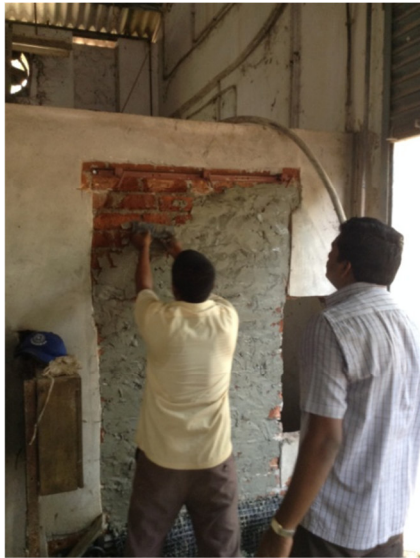
(c) Application of first layer of FABmix
