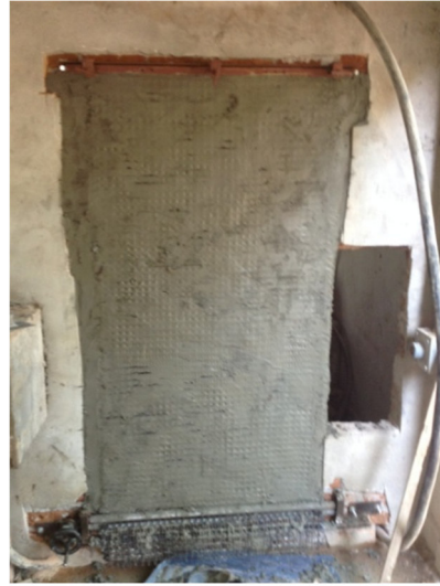
(g) Application of final layer of FABmix (h) After application of final layer of FABmix
