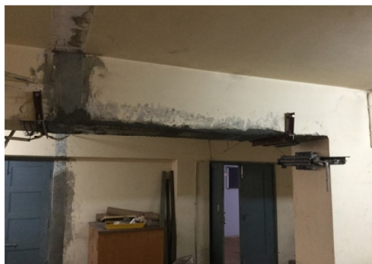
(h) Beam after application of TRC
