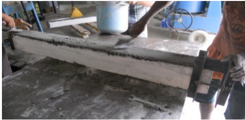
Applying final layer of FABmix
