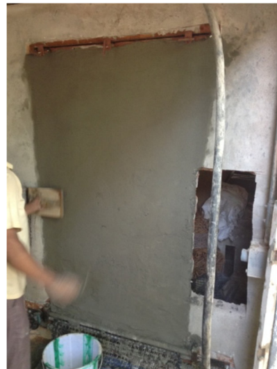
(i) Levelling of final layer of FABmix
