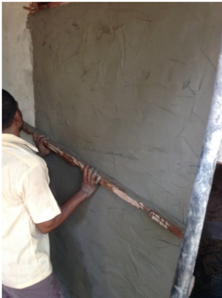
(i) Levelling of final layer of FABmix
