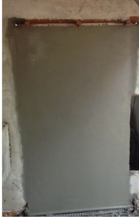
(j) Masonry wall after application of TRC
