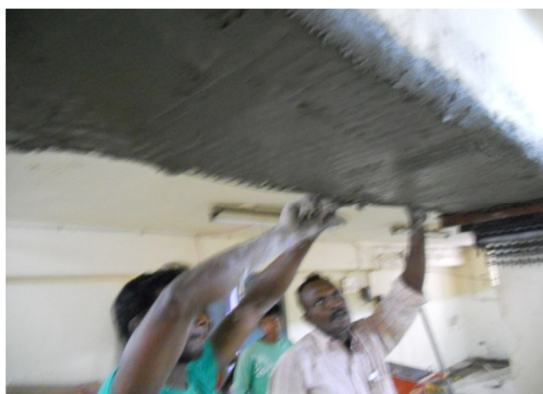
(g) Application of final layer of FABmix
