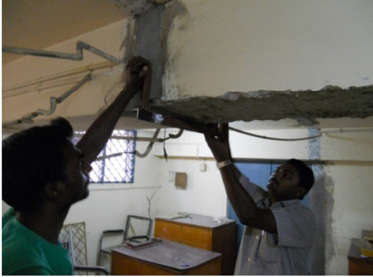
(a) Fixing the non-stretching unit in beam
