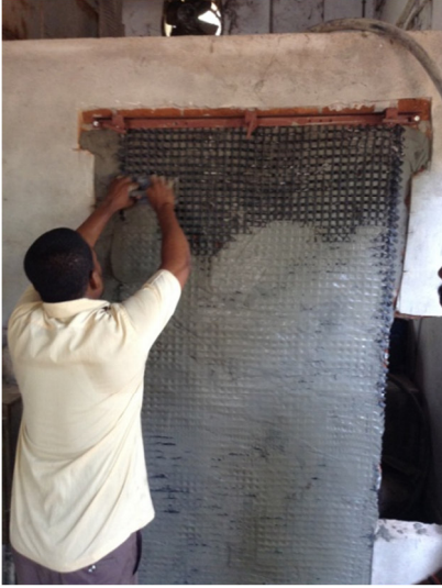
(g) Application of final layer of FABmix (h) After application of final layer of FABmix
