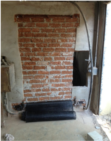
(a) Tautening apparatus fixed in the wall
