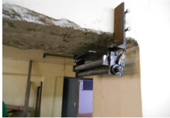
(b) Fixing stretching unit in beam
