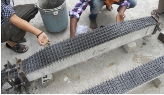
Applying first layer of FABmix
